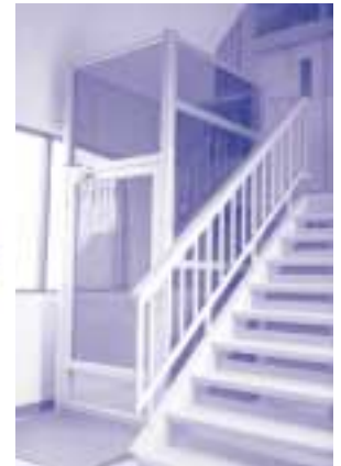
Figure 12: Vertical lifts are often installed next to a set of stairs. Courtesy of Garaventa Accessibility
