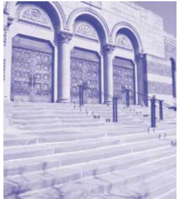
Figure 3: This synagogue's steps and massive doors are not only insurmountable for those in wheelchairs, but also for many elderly congregants. Neal Vogel for Restoric, LLC
