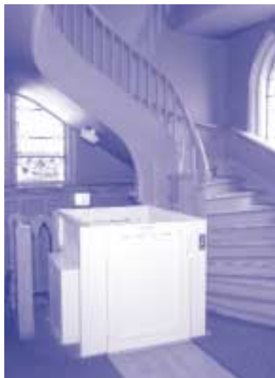
Figure 4: Custom enclosures are usually required to minimize the aesthetic impact of lifts in historic settings. Michael Schmidt for Restoric, LLC
