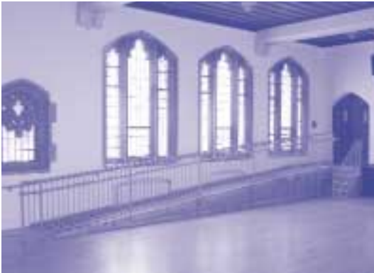
Figure 9: This interior ramp improves ALL traffic flow between the original church and a parish house addition. Michael Schmidt for Restoric, LLC
