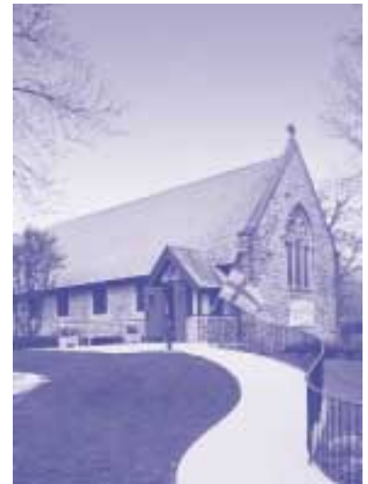
Figure 5: At this entrance, a small stoop was replaced with a bermed walk and landscaping to create accessibility. Neal Vogel for Restoric, LLC
