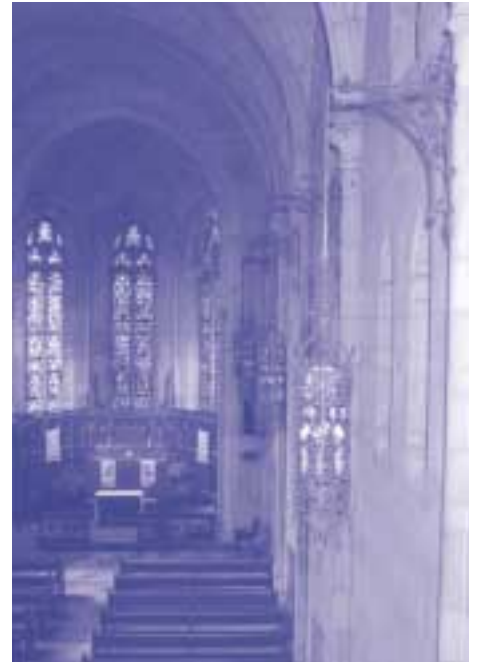
Figure 15: These beautiful historic light fixtures were not designed to meet modern lighting standards but should be preserved by utilizing supplemental lighting as required. Michael Schmidt for Restoric, LLC
