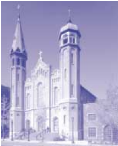
Figure 11: A lift installation (behind the right steeple) proved to be an economical and aesthetically pleasing alternative to a massive ramp on the front of this historic church. Courtesy of Booth Hansen Associates
